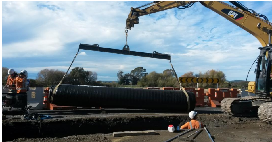
Havelock North Relief Sewer Construction on SH2
