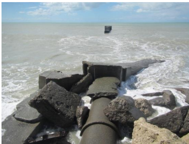
Emergency Beach Overflow Structure
