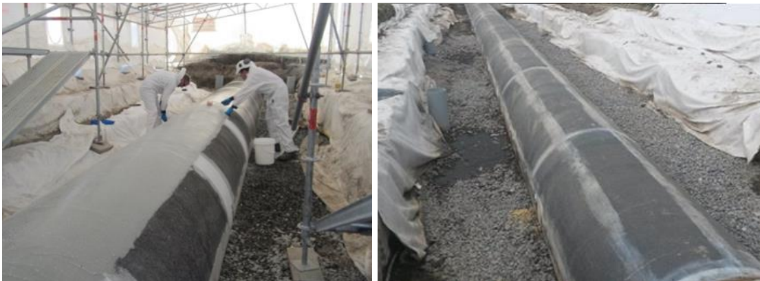
Repair of Landward Section of the Outfall Pipe
