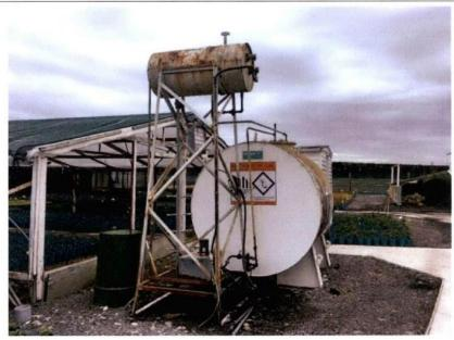
Plate 3: The existing oil tank and hand pump, visible on the ground beneath the hand pump is a small area of hydrocarbon contamination.
