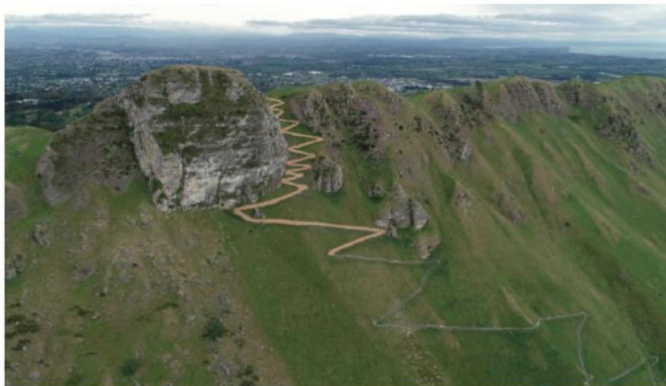
Figure 4: Drone Photograph of coconut (BioCoir) matting covered emergency works from south east 9/11/2018
