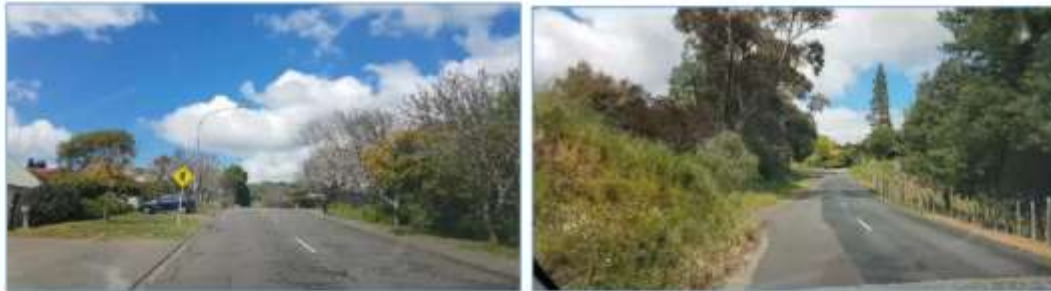
Figure 3-15: Road surface Condition – Alligator Cracking on Simla Avenue (left) and flushing on Te Mata Peak Road (Right)
