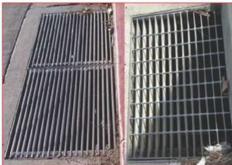
Figure 4-13: Example of Cycle Friendly Stormwater Grates
