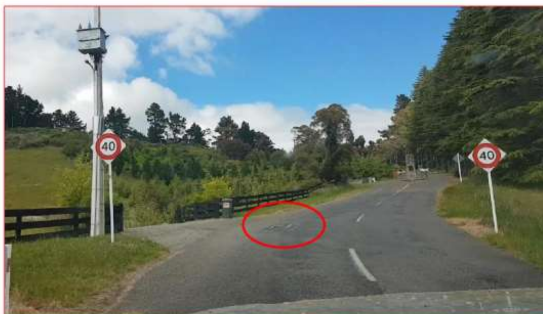
Figure 5-2: Inconsistent Posted Speed Limits between Roadside Markings and Signage
