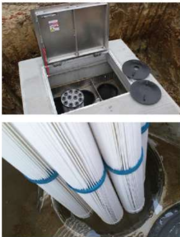
Figure 6.7: Stormwater 360 Jellyfish Unit
