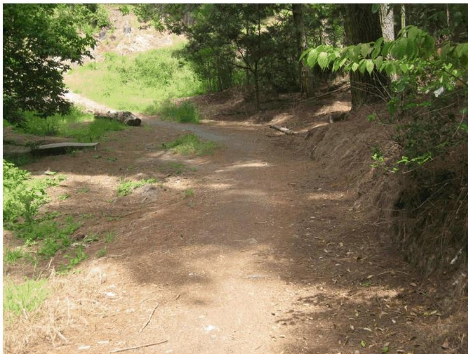
Fine leaf litter will aid the binding of an aggregate surface over time
