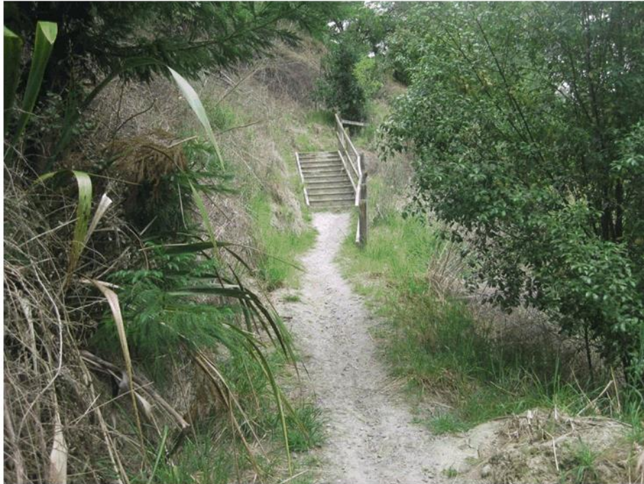
Sections of steps can often be avoided by simply adjusting the track alignment
