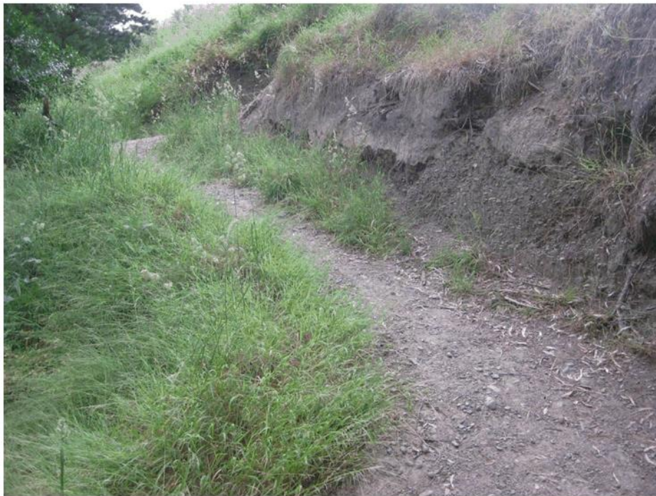
Tracks at the base of slopes should be provided with a side drain
