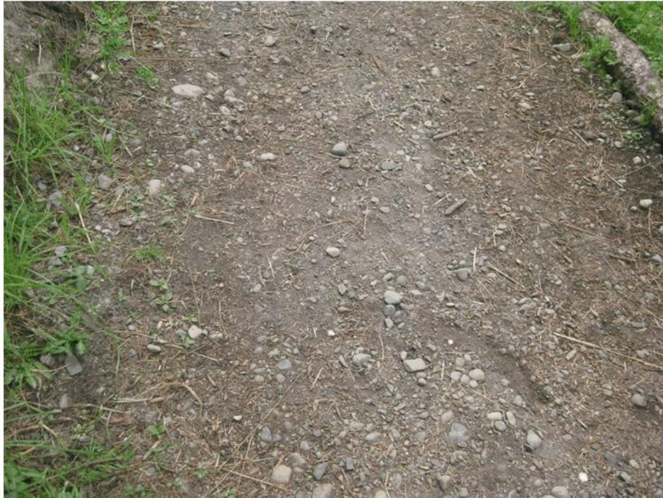
Rounded gravel path surfacing aggregate will not bind
