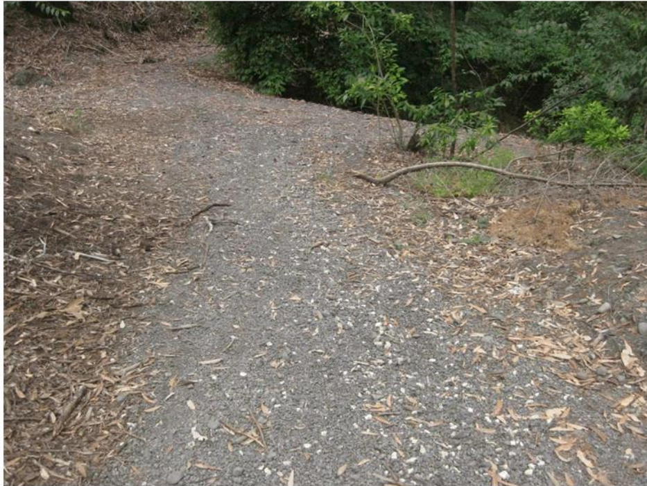
Pea gravel does not provide a stable track surface, and can be dangerously slippery
