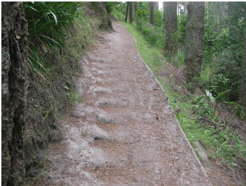
Steep sections of track need to be re-routed or have proper steps installed
