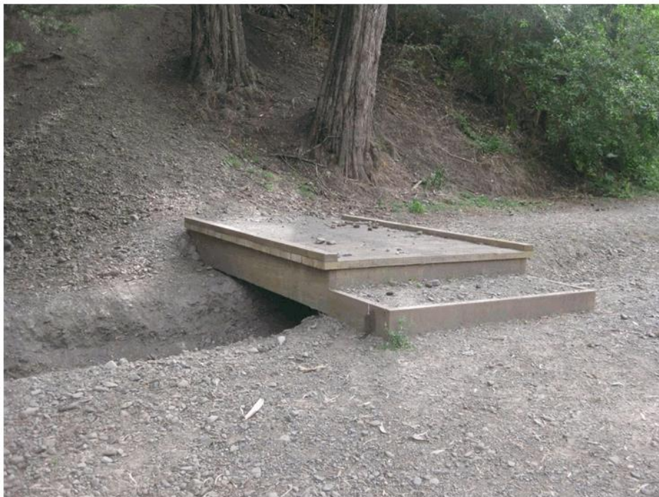
Avoid steps onto boardwalks. These are barriers to cycles and push-chairs
