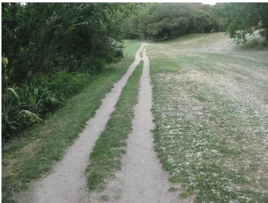
Track on low areas could be raised slightly to provide drainage
