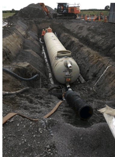
Installation of Omahu Industrial wastewater storage chamber and pump station.
