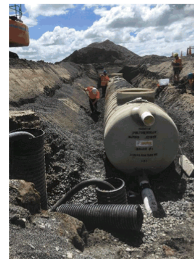
Installation of Omahu Industrial wastewater storage chamber and pump station.
