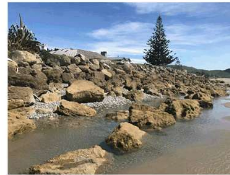
Figure 4 – Seawall in Acceptable Condition, Voids Require Filling
