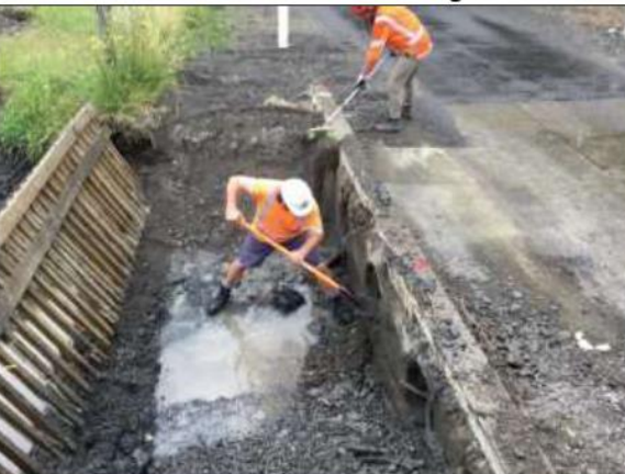
Soldiers Settlement Road: Culvert Cleaning
