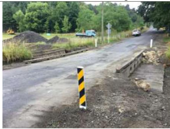
Soldiers Settlement Road: Culvert Cleaning
