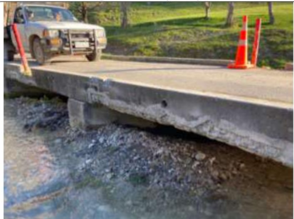
Mackenzie Rd: Bridge Concrete spall repairs
