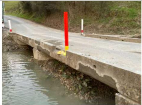
Mackenzie Rd: Bridge Concrete spall repairs
