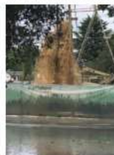
FLUSHING OF THE BORE
