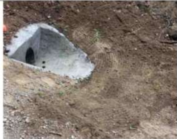
Flat Hill Rd: Headwall Construction
