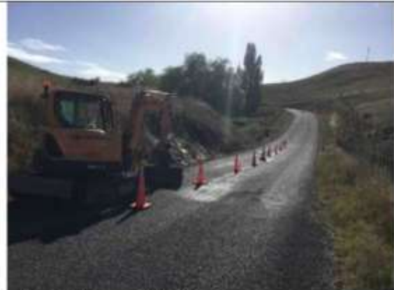
Taihape Rd: Watertable Maintenance
