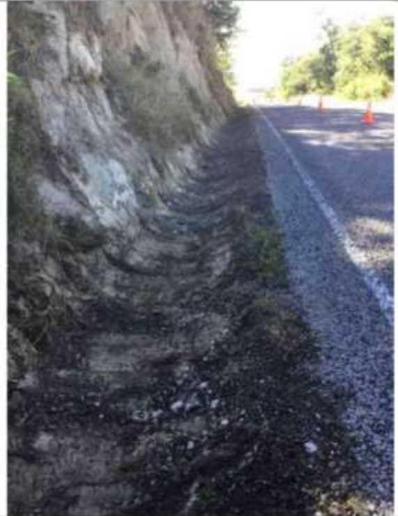
Taihape Rd: Watertable Maintenance
