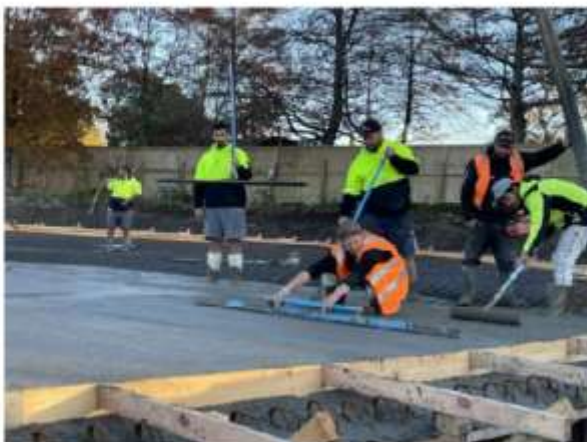
Second tank foundations
