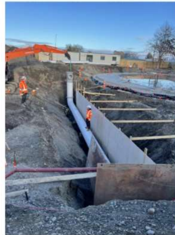
Scour pipe installation
