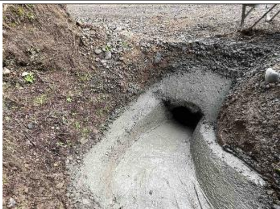
Glenbrook Rd: Culvert Maintenance
