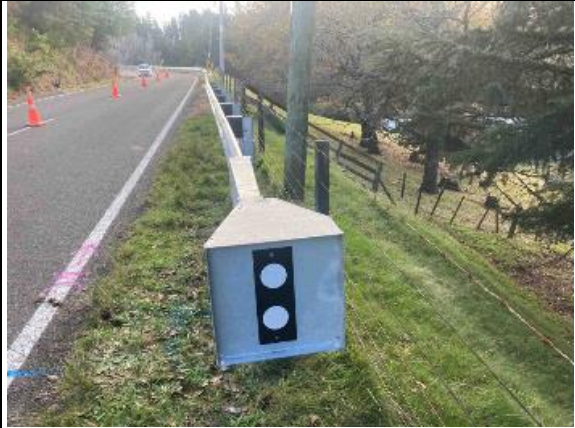
Taihape Rd: Guard Rail Installation
