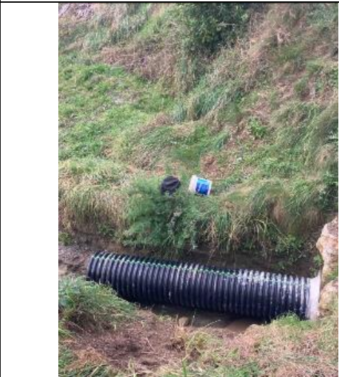
Huiarangi Rd: Culvert Extension
