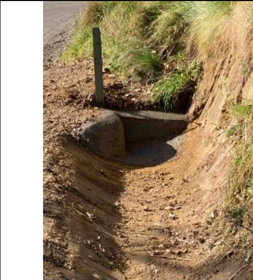
Huiarangi Rd: Culvert Extension
