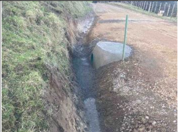
Mokamoka Rd: Headwall Installation
