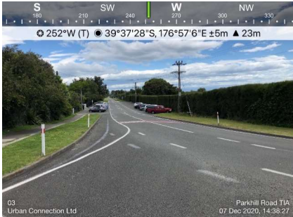
Figure 25: Sight distance to the west at the Parkhill Road/Raymond Road intersection
