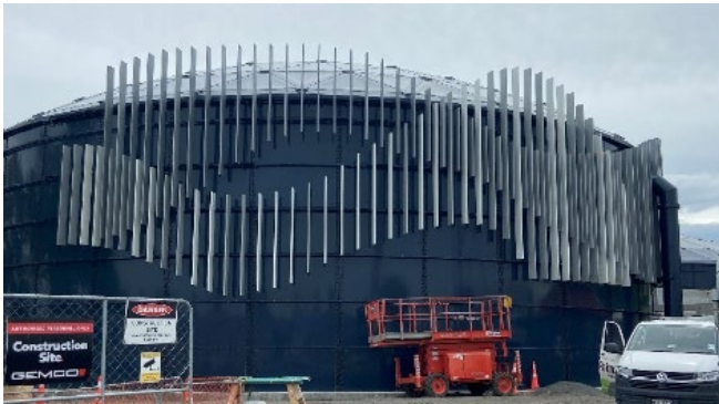
Southern tank Architectural Fin installation
