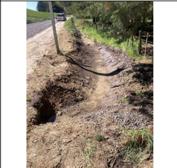
Te Apiti Rd North: Drop Out Repair
