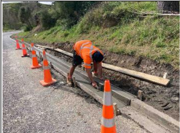
Waimarama Rd: Kerb & Channel Installation
