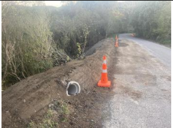
Willowford: Culvert Installation
