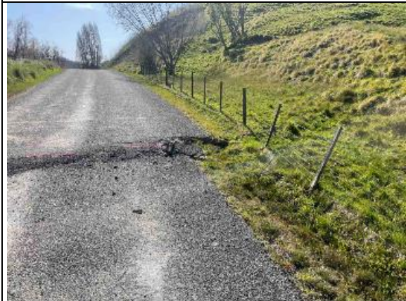
Te Apiti Rd North: Drop Out Repair
