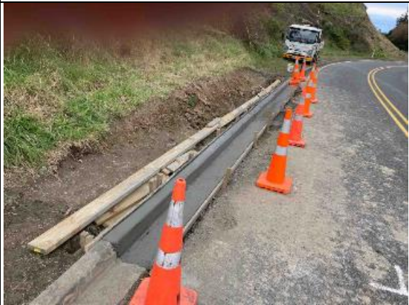
Waimarama Rd: Kerb & Channel Installation
