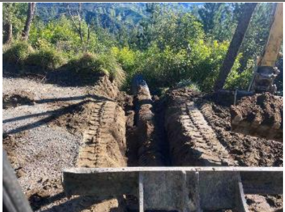
Pohokura Rd: Culvert Installation
