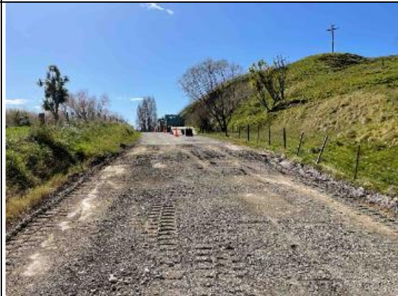
Te Apiti Rd North: Drop Out Repair
