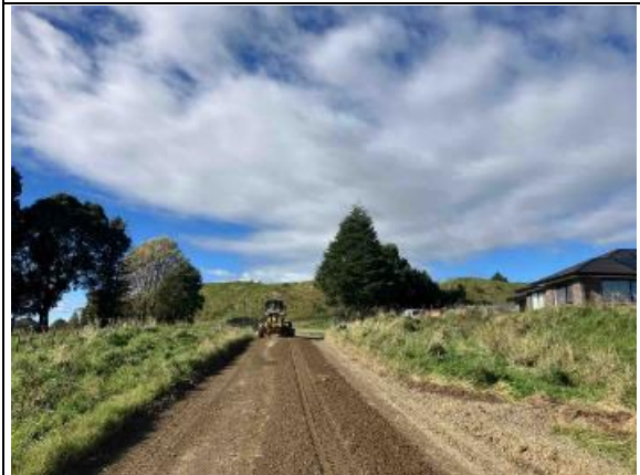
Kahuranaki Rd: Dropout Repair
