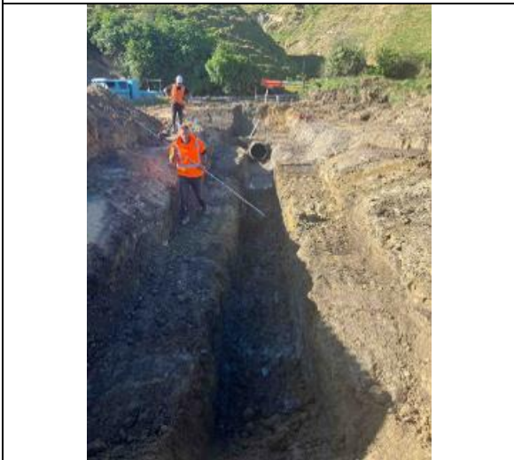
Maraetotara Rd: Culvert Installation
