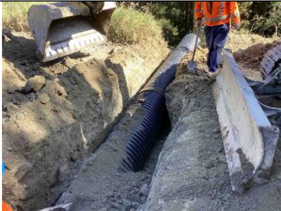
Pohokura Rd: Culvert Installations
