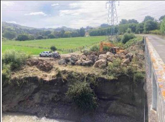
Waipunga Rd: Bridge Scour Repair
