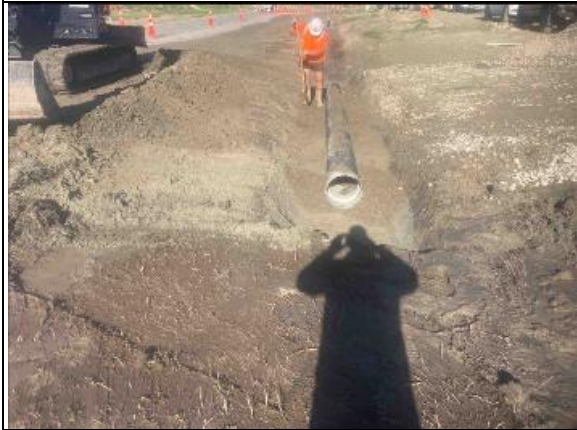
Tangoio Settlement Rd: Culvert Installation
