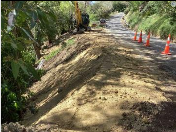
Kahuranaki Rd: Dropout Repair
