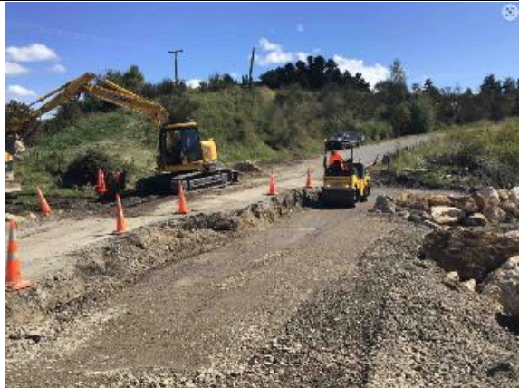
Salisbury Rd: Washout Repair
