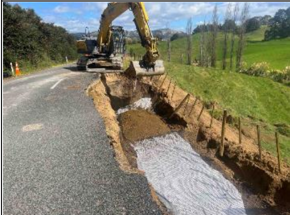
Matahorua Rd: Dropout Repair
