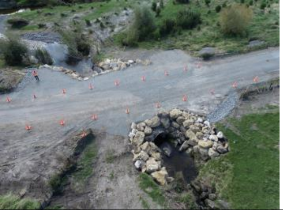
Salisbury Rd: Washout Repair
