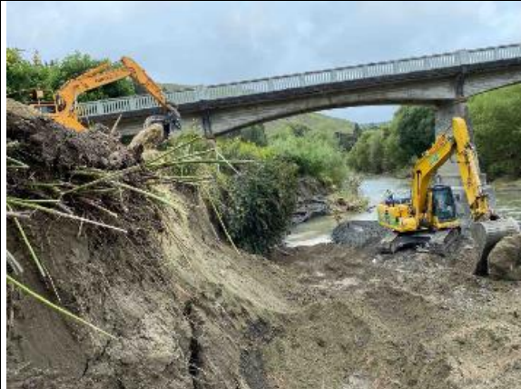
Waipunga Rd: Bridge Scour Repair
