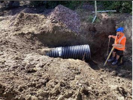
Pohokura Rd: Culvert Installations
