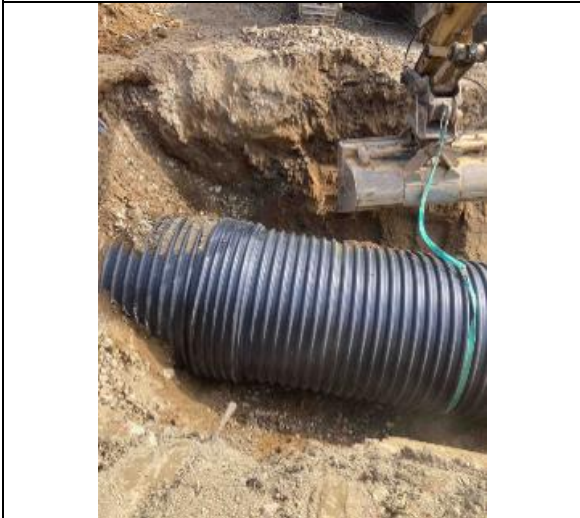
Pakaututu Rd: Culvert Installation
