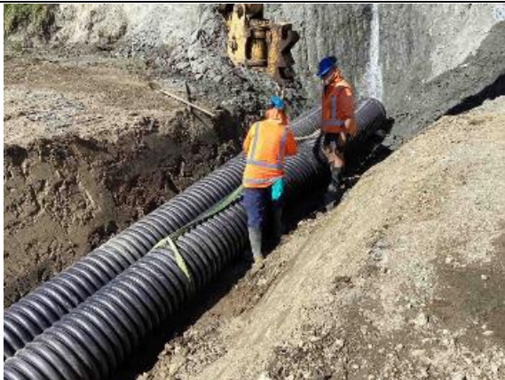
Pohokura Rd: Culvert Installations
