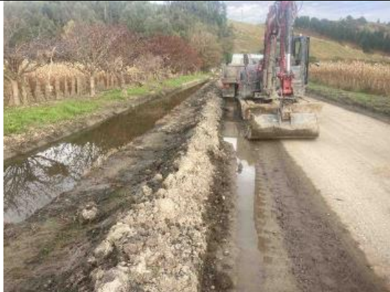
Pohokura Rd: Culvert Installation
