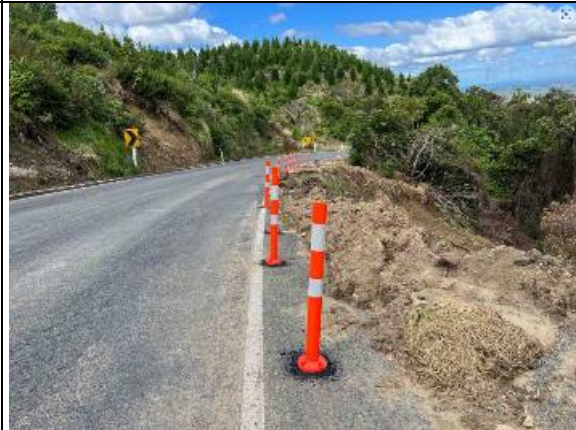
Taihape Rd: Bollards Installed
