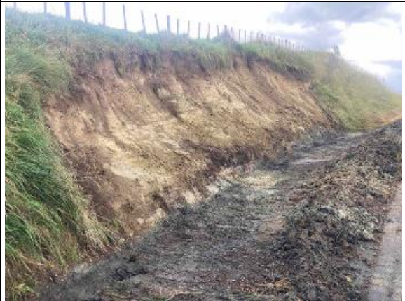
Otamauri Rd: Dropout Repair
