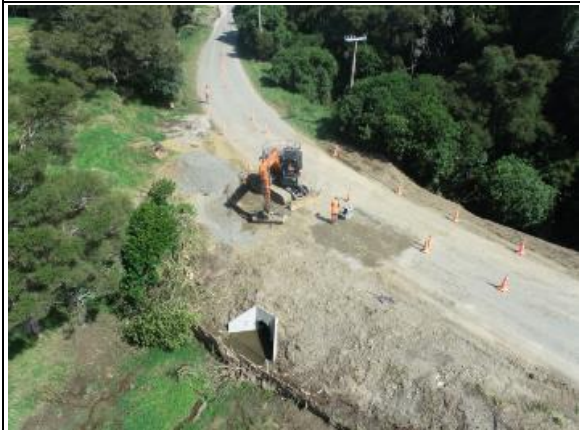
Pakaututu Rd: Culvert Installation
