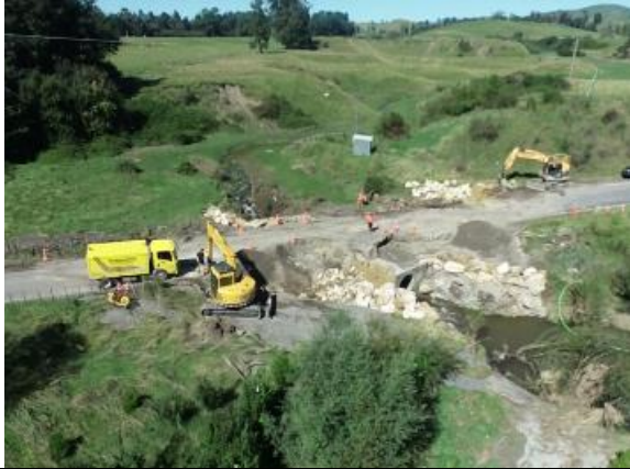
Salisbury Rd: Washout Repair
