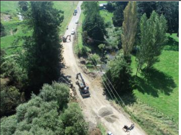
Dartmoor Rd: Clearing Culverts
