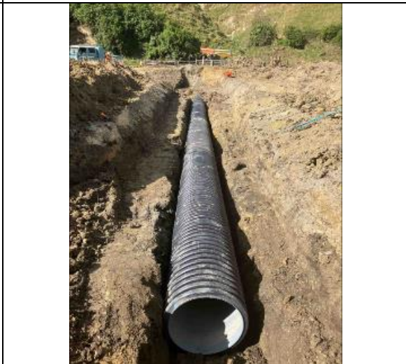
Maraetotara Rd: Culvert Installation
