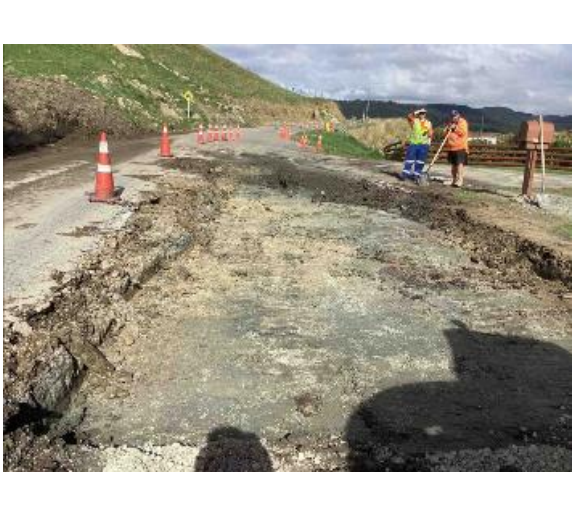
Dartmoor Rd: Stabilization Dig Out
