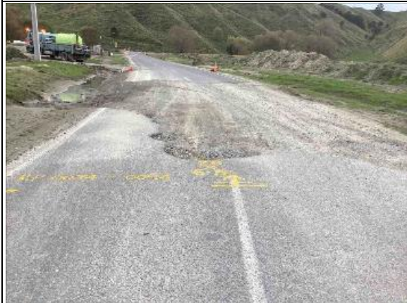
Tangoio Settlement Rd: Culvert Installation
