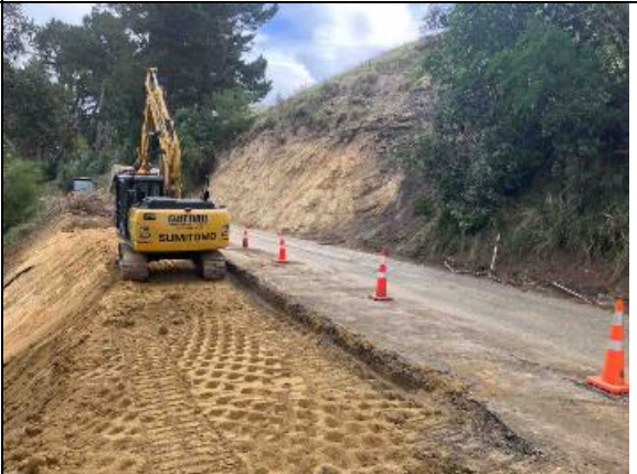
Matahorua Rd: Dropout Repair
