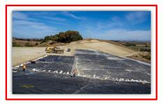
HDPE (plastic) and GCL (geosynthetic clay liner) being installed in Stage 3A of Area D
