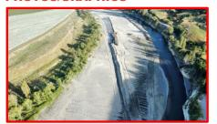
Work diverting the Tūtaekuri River in order to repair slip 7.69
