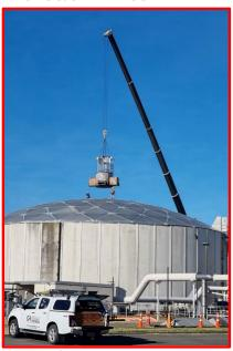
Installation of BTF distribution arm central column at East Clive WWTP
