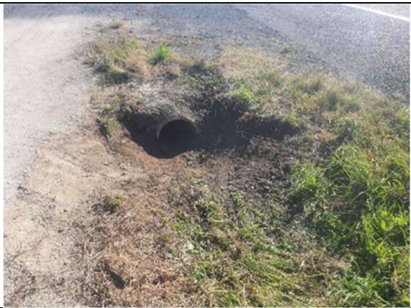
Maraekakaho Rd W: Broken Headwall Removal
