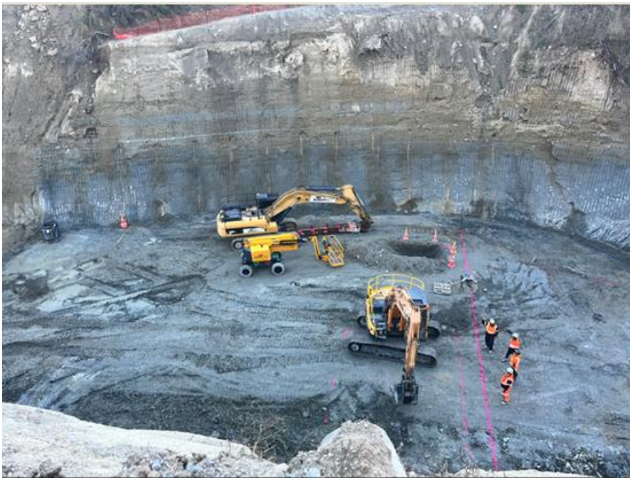
Photo: Section being marked out before soil mixing (11 June 2024).
