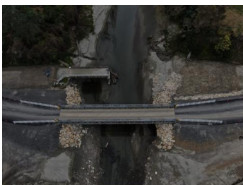
Photo: Image of the old Whanawhana Bridge and temporary bailey bridge.
