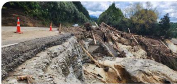
Large underslip at Captain's Culvert
