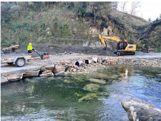
Photo: Repaired McIntyres Low-Level Crossing with culverts,
