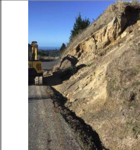
Aropaoanui Rd: Slips Clearing
