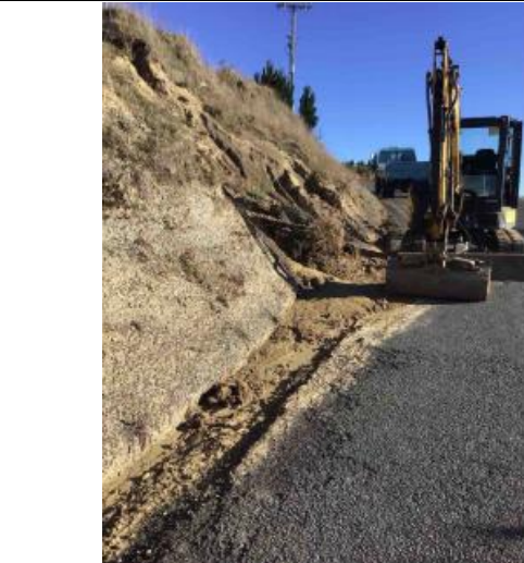
Aropaoanui Rd: Slips Clearing
