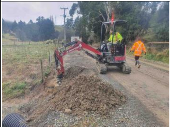
Waikoau Rd: Dropout Repair
