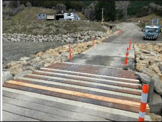
Aropaoanui Rd: Bollard Installation
