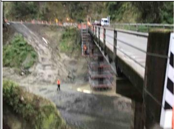
Waikoau Rd: Waikoau Gorge Bridge: Scaffolding Installation
