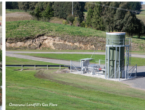
Omarunui Landfill's Gas Flare
