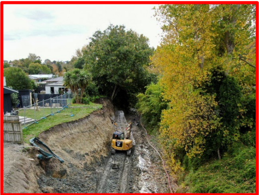
Tri-party bank solution on the upper Mangarau Stream, under construction
