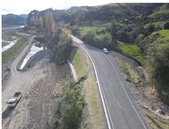
After: Reinforced earth wall and new 2.1m culvert with rip-rap protection.
