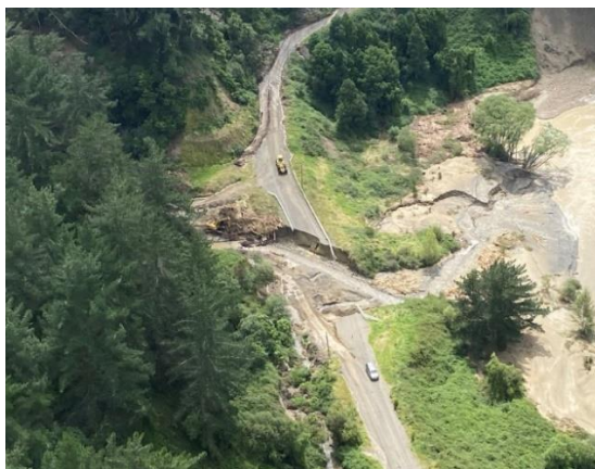
Aerial image of McVicars Culvert damage
