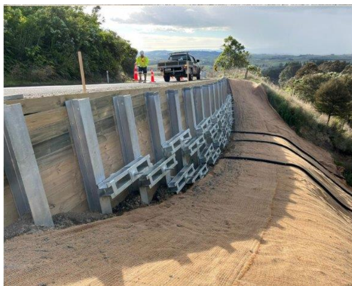
Consisted of four under slips in proximity. Fix involved building four steel piled anchored retaining walls, stormwater improvement and lengthening the existing guardrail.
