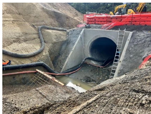
First of its kind fish ramp designed in collaboration with mana whenua, ecology and WSP consultants to accommodate safe passage through the culvert fish.
