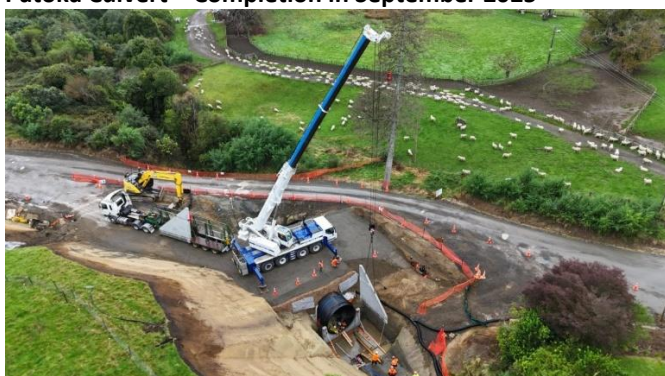
Culvert washout. Utilised repurposed pipe from Chrystal Twin Culvert.
