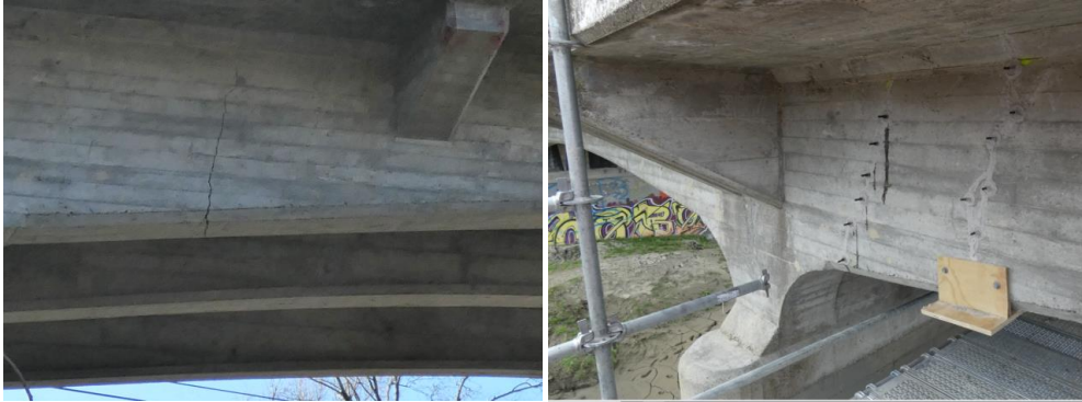
Figure 14: Cracks in Beams of Existing Bridge (3 rd span from Napier) Before (Left) and After (Right).
