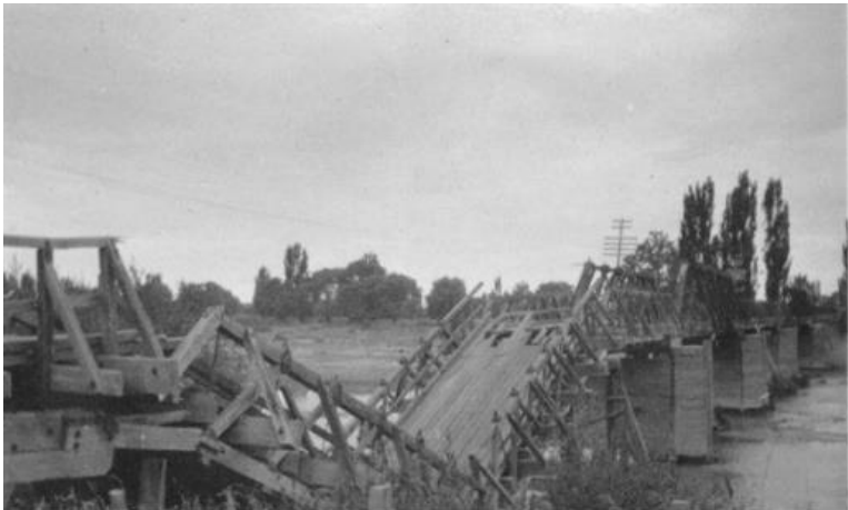
Figure 4: Original Bridge after 1931 Earthquake from NZSEE Paper 3
