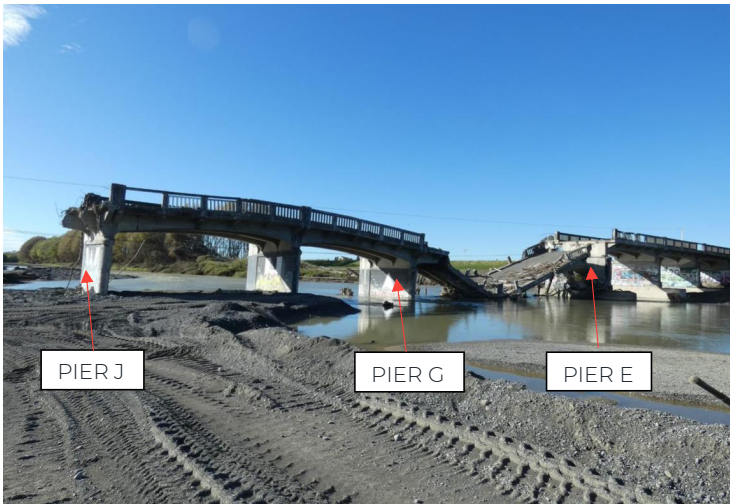
Figure 7: Redclyffe Bridge damage after Cyclone Gabrielle
