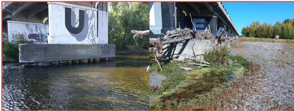
Figure 4: Potential scour around piers prior to 2023 Cyclone event.
