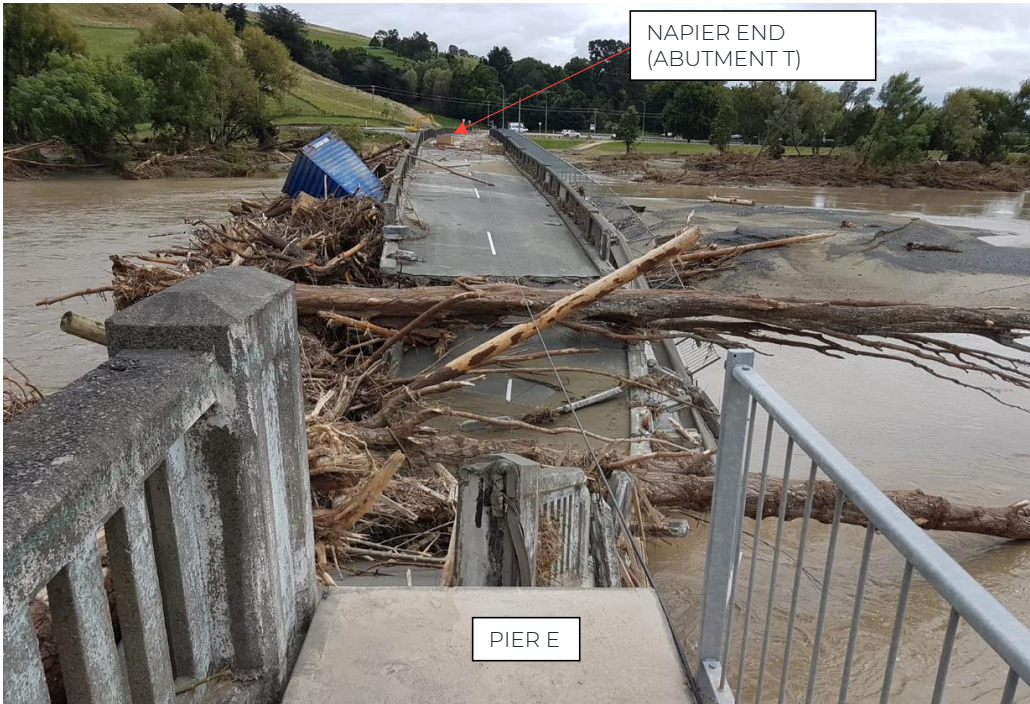
Figure 5: Redclyffe Bridge damage after Cyclone Gabrielle
