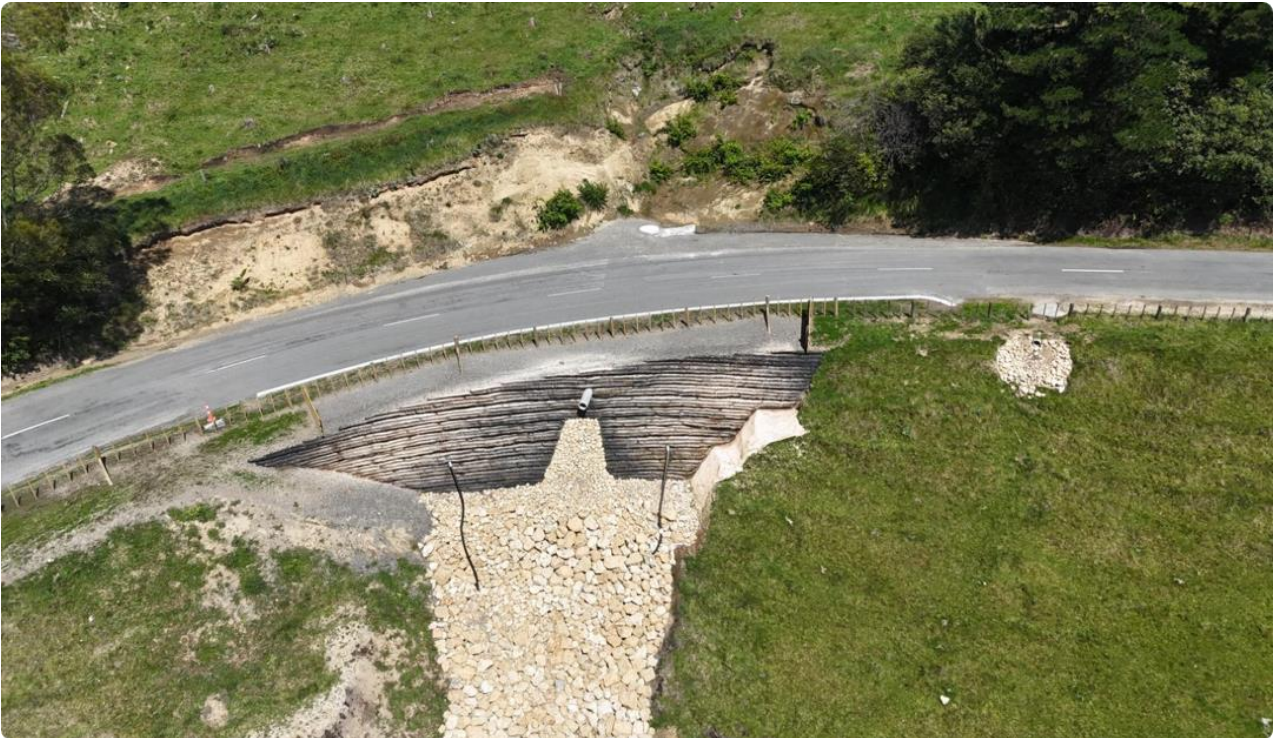
A large slip on Matahorua Road (north of Tutira) was reinforced to protect the existing road from further erosion.
