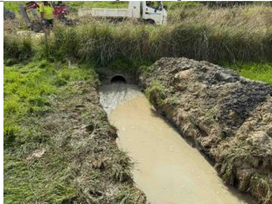
Okaihau Rd: Watertabling and Flushing
