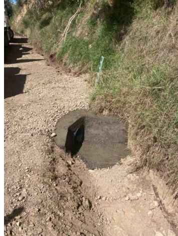
Maraetotara Rd: Watertabling & Headwall Install
