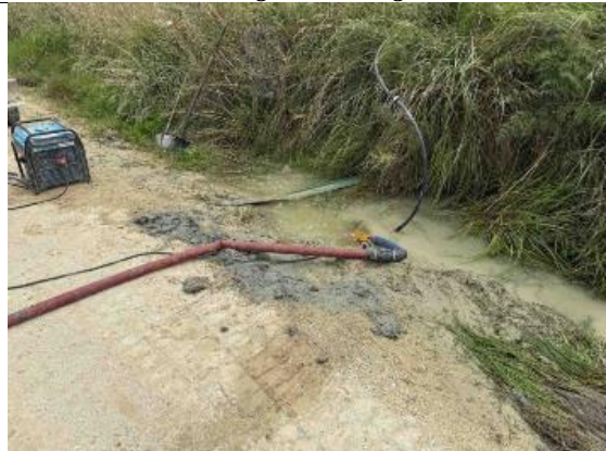
Okaihau Rd: Watertabling and Flushing
