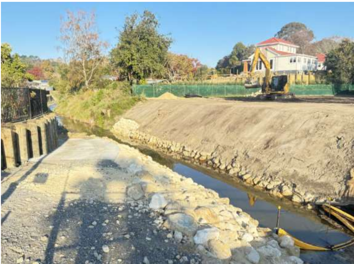
Figure 4: Stage 2 works under construction at 4 May 2026
