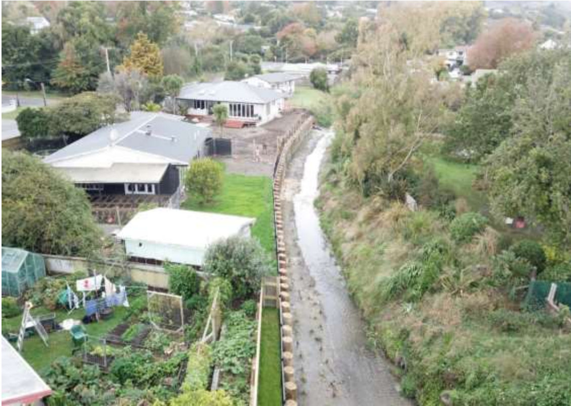
Figure 1: Work in progress on Stage 1 - Seperable Portion 1 – Bank Remediation 13 April 2026
