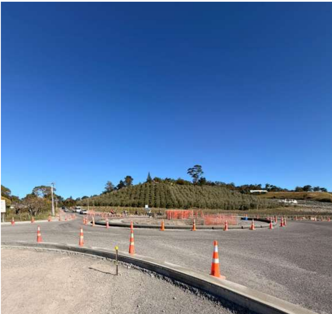
Figure 3: Te Mata/ Waimaramā Roundabout
