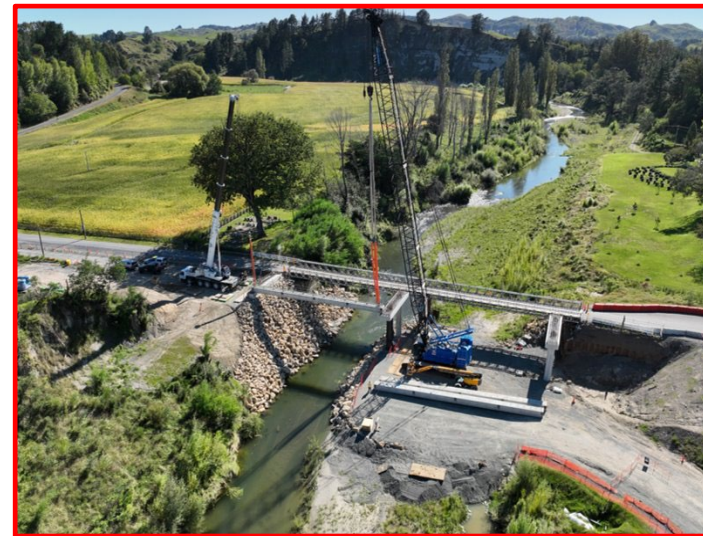
Rissington Bridge rebuild, beam installation
