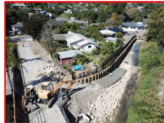
Plassey Street – Stage 1 Completed Access Ramp
