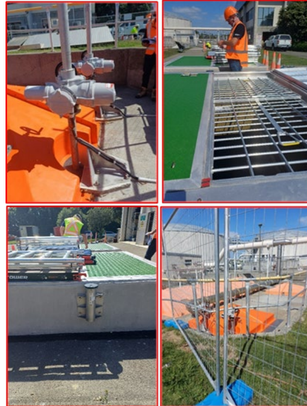
WW Picture: Recently upgraded and commissioned WWTP Penstock at East Clive
