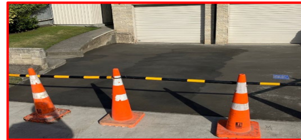
SW localised improvement completed by raising the driveway at 105 Ballantyne Street
