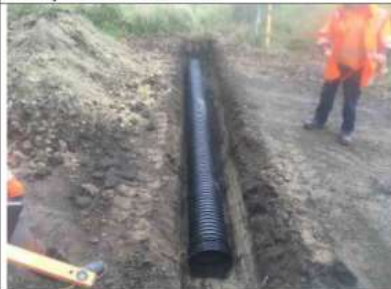
Wenley Rd: Culvert installation
