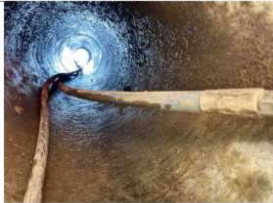
Hawkston Rd: Watertabling and culvert flushing
