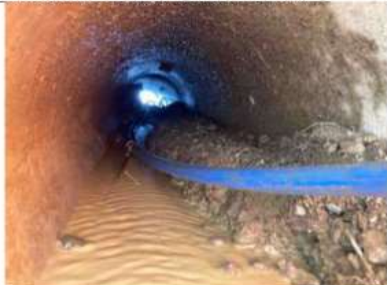
Hawkston Rd: Watertabling and culvert flushing
