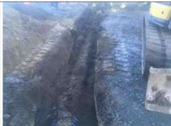
Little Bush Rd: Culvert installation
