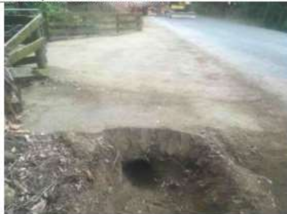
Hawkston Rd: Watertabling and culvert flushing
