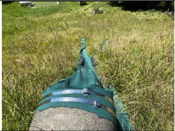
Seafield Rd: Sock Installation
